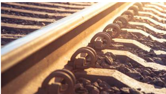
E-clip railway fastening system
